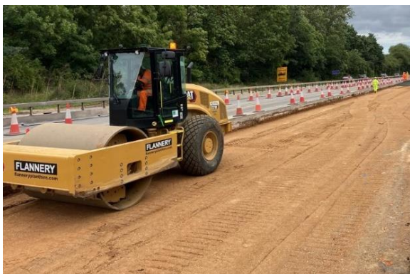
A roller making sure the ground is level
