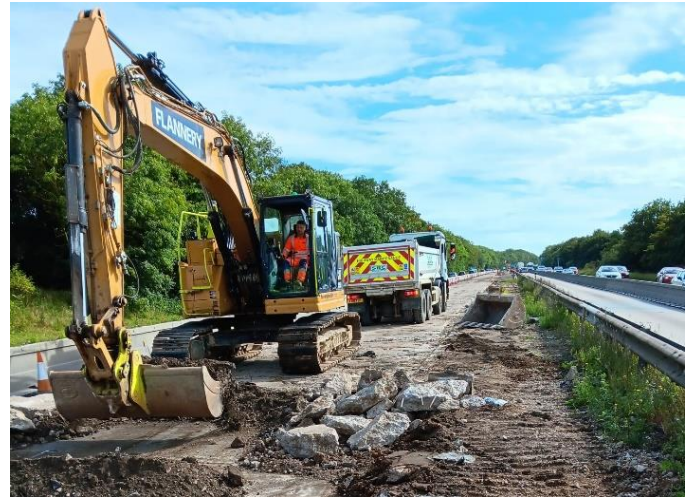
Concrete foundations being removed
