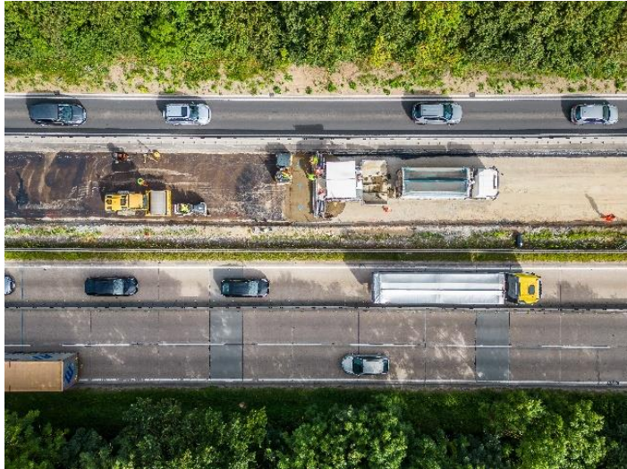
A bird's eye view of the A12 northbound work
